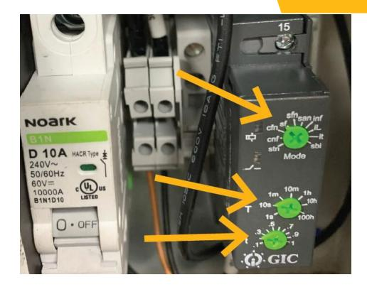
Mode: sf (signal off delay – Délaie de désactivation)
